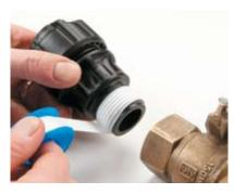
Apply PTFE tape or suitable\* sealant to the plastic thread ensuring sufficient is applied to ensure a watertight seal.
