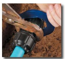
5. Nut Tightening The nut should be tightened firmly with multi-grips or similar plumbing tools until the nut just touches the flange on the body of the fitting.
