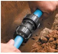
**5. Pipe Insertion**Insert the pipe fully into the fitting to the point where the stop is felt.
