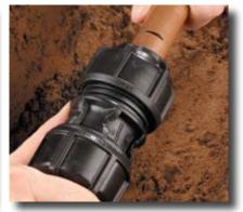
Pipe Insertion Insert the pipe fully into the fitting up to the witness mark.
