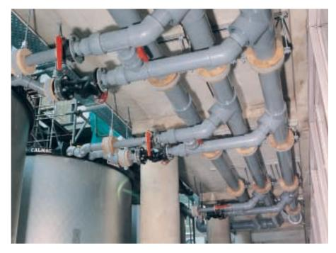
The corrosion resistance of the piping material is as important since the aqueous solutions used by such systems may be of a corrosive nature. These have highlighted the benefit of the corrosion resistance of Durapipe ABS piping systems. Growing economical and environmental pressures have also made Durapipe ABS piping the right choice.
