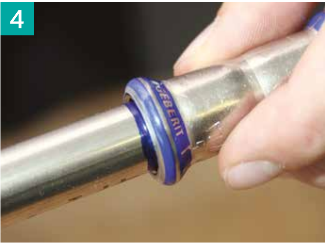
INSERT PIPE INTO FITTING
