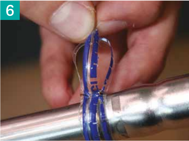
REMOVE PRESSING INDICATOR
